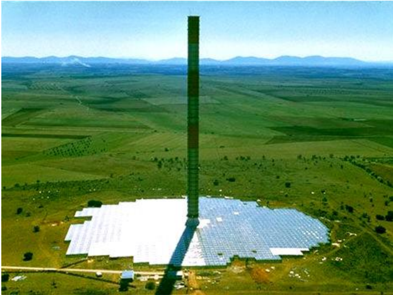
Prototype 50 kW solar tower in Manzanares, Spain, 1982-1989 ( Enviromission ).
